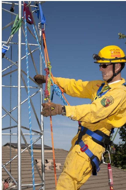
Figure 14-5. Victim lowering attachment points.
