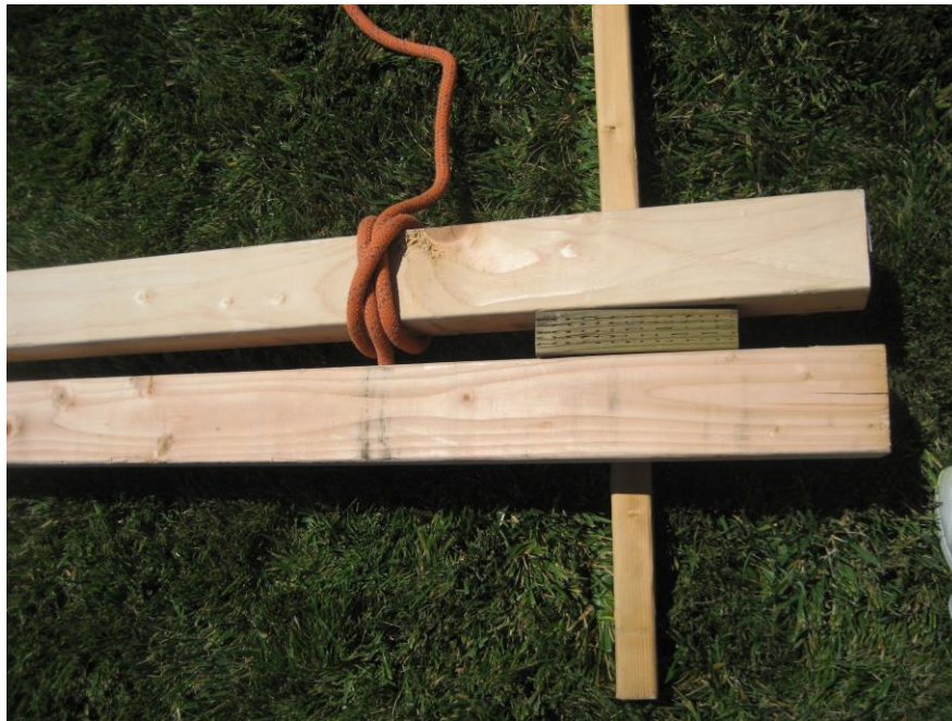
Figure 16-5. Clove hitch on one leg.
